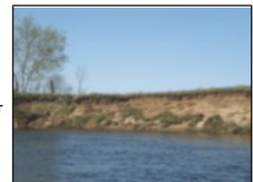
Bank erosion along the Rum River.
