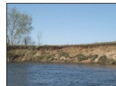
Example of erosion along the Rum River identified during a spring 2010 field survey.
